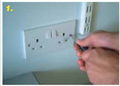
1. Undo screws and pull face plate forward 5mm
