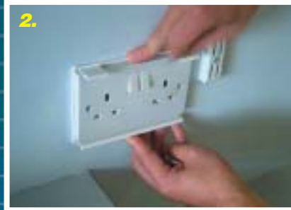
2. Fit Plug Lock rear frame
