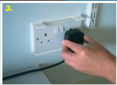
3. Tighten screws and fit appliance plugs
